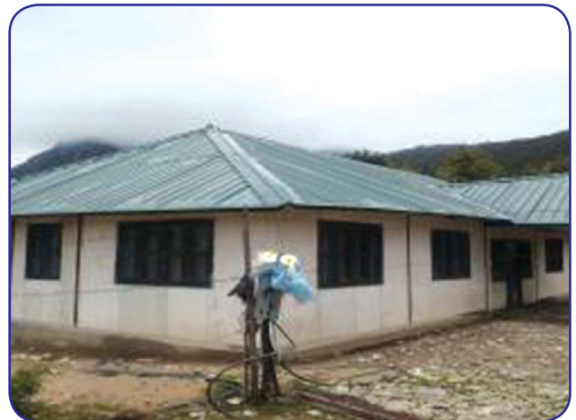
चित्र ८: Prefab building construction at Namche
